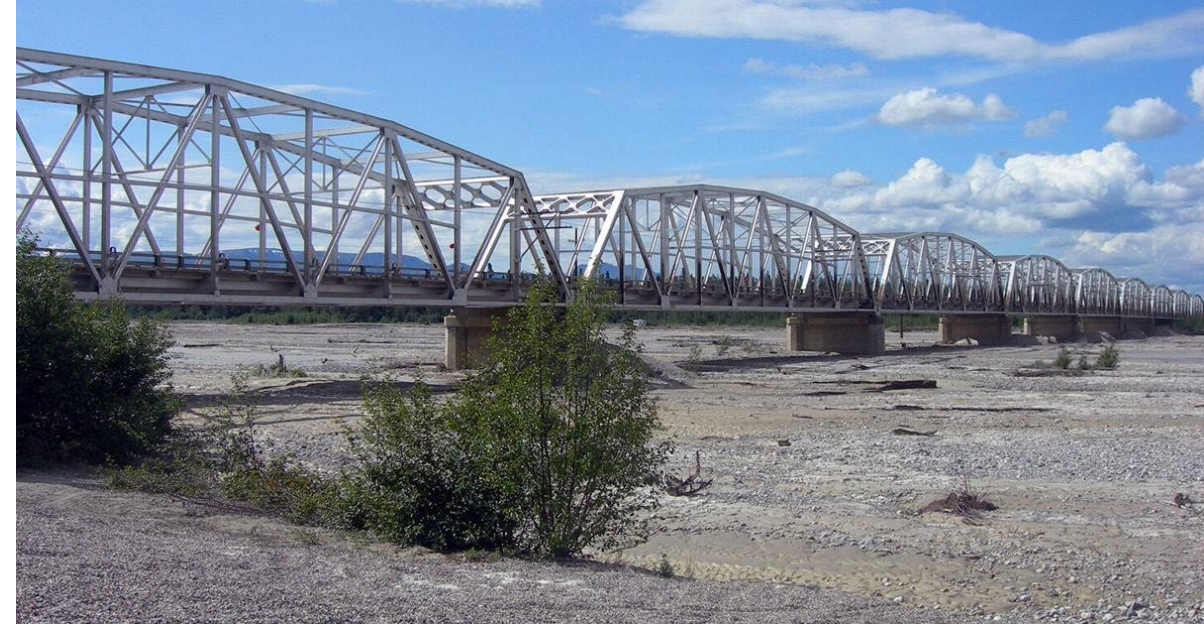
Gerstle River Bridge, AK
