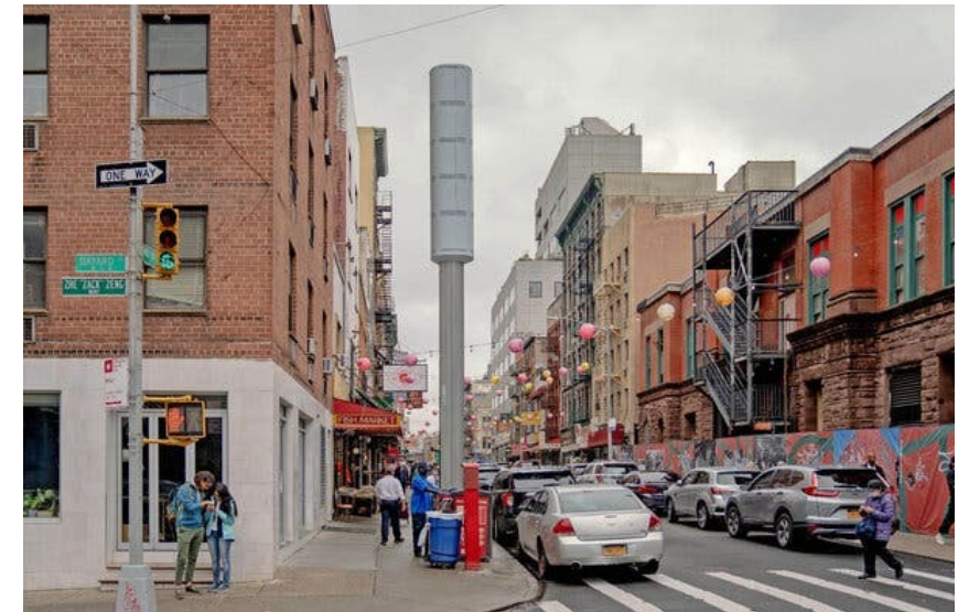
5G Cell Towers, Phoenix and New York City
